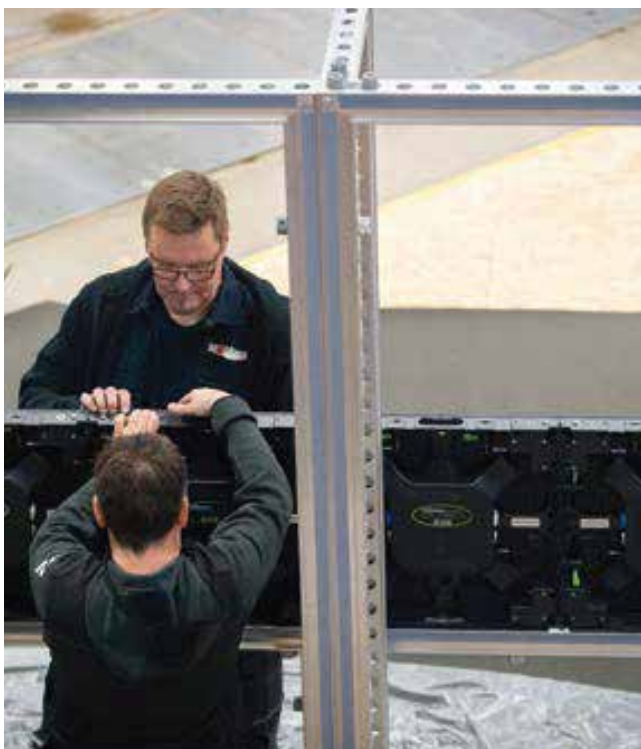
Fixing the LEDskin™ frames to the beMatrix aluminium frames is easy with the handy standard M8 connectors. Ready in a jiffy and always firmly and securely anchored.
